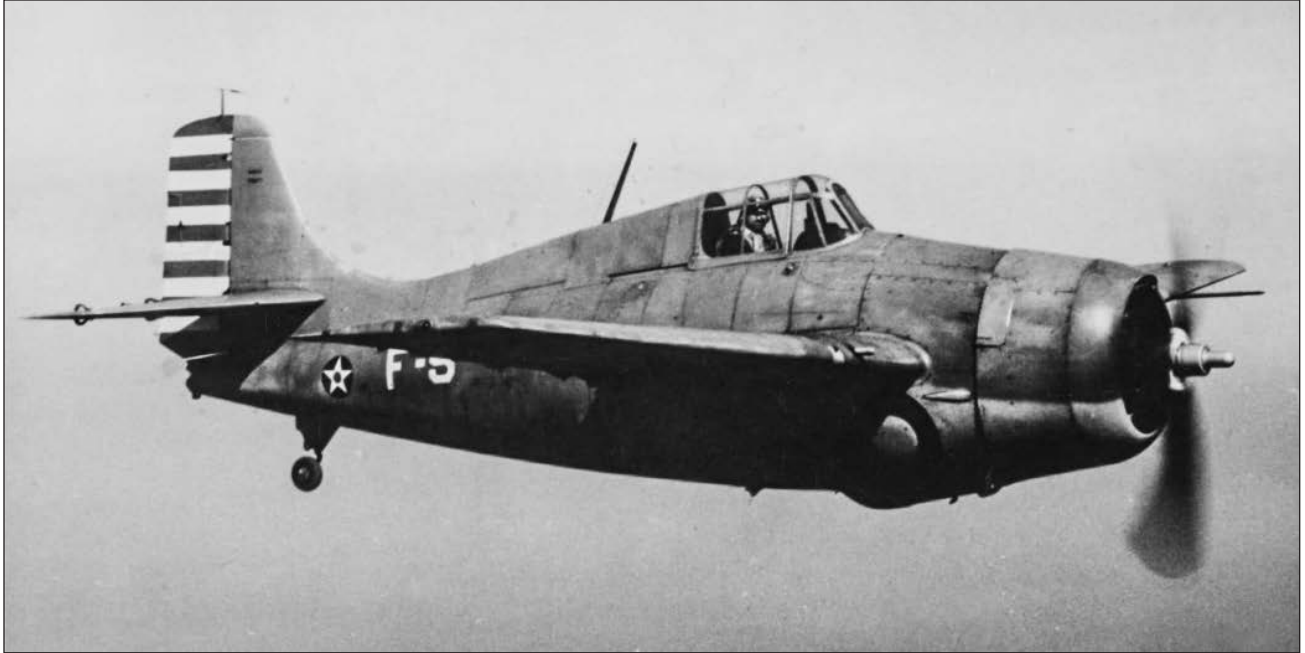
In the Coral Sea, the Lexington and Yorktown were equipped with this (F4F-3) version of the Grumman "Wildcat" fighter. At that time the red center circle of our star insignia and red and white horizontal tail stripes had not been eliminated. The rugged F4F-3 was outflown but not outfought by the "Zero," having superior armament and carrying both armor and self-sealing gas tanks.
